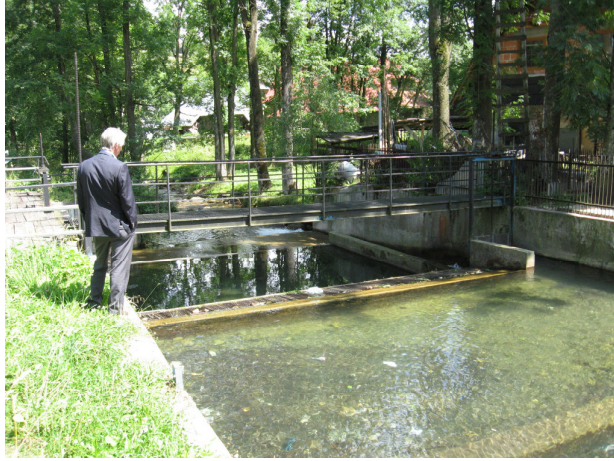
Figure 7 The author admires the flow through an supply channel for a power plant in the Polish Mountains'
