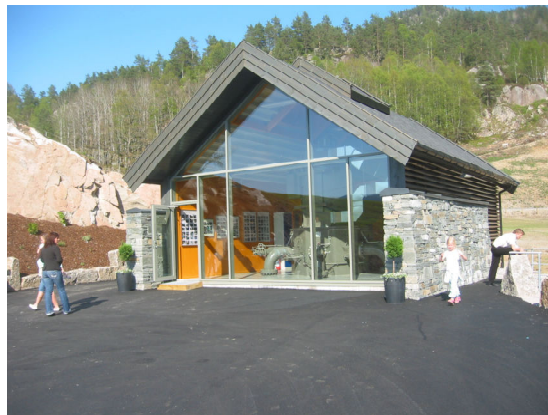
Figure 2 Oftedal Small Hydro Power Plant (Norway) 2006
