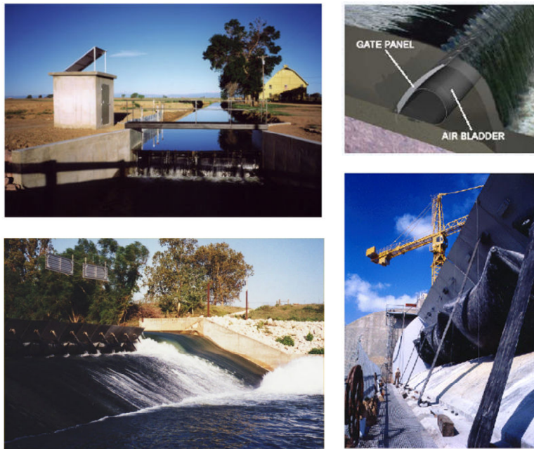
Figure 4 Pneumatic operated Spill Gates forming the dam
